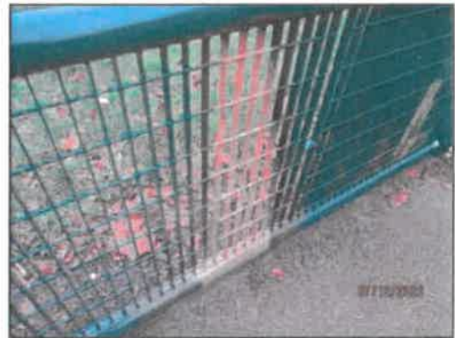
(Slight fire-damage to panel)
