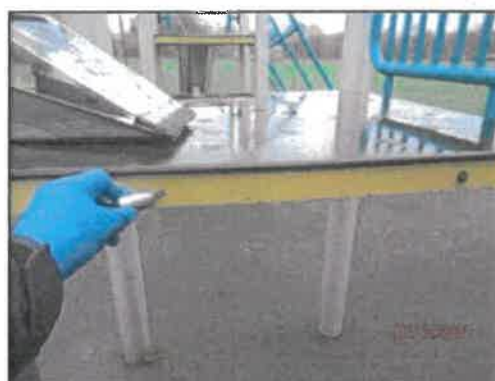
(Potential finger trap at missing bolt)
