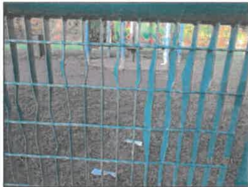
(Slight damage to mesh panel – library photo)
